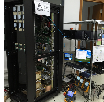
Fig. 8 The 110V-5kVA SVC-HAPF experimental prototype and its testing environment
